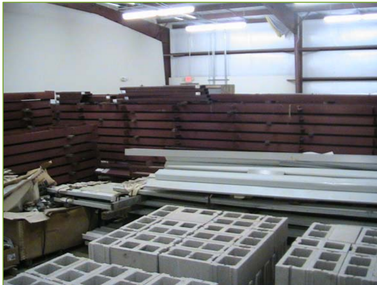
On Site Nucor Steel Buildings Awaiting Assembly
